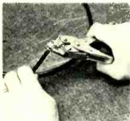
7. Crimp sleeve with crimping tool, pinching drain wires tightly.
