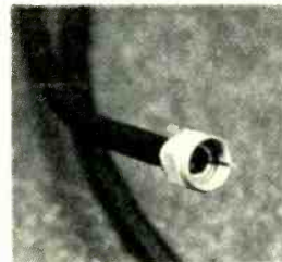
9. Coat finished connector with silicone grease inside and out for weatherproofing.
